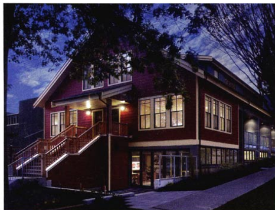
A heritage Vancouver schoolhouse attains new life as an eye-catching condominium renewal project by Trillium Project Management.
